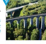
Built in 1866 to carry the Brecon and Merthyr railway across the river Taff, this majestic viaduct has 15 arches each one is 39ft 6ins wide. The last passenger train passed over the viaduct in 1964 after which it fell into disrepair.
