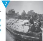
onstructed 1790 - 1794 the canal was designed by Thomas Dadford for Merthyr's Crawshay Ironmasters, to transport iron from Merthyr to Cardiff as quickly and as cheaply as possible. It covered over 25 miles with 51 locks having to be made to allow for the 543ft
